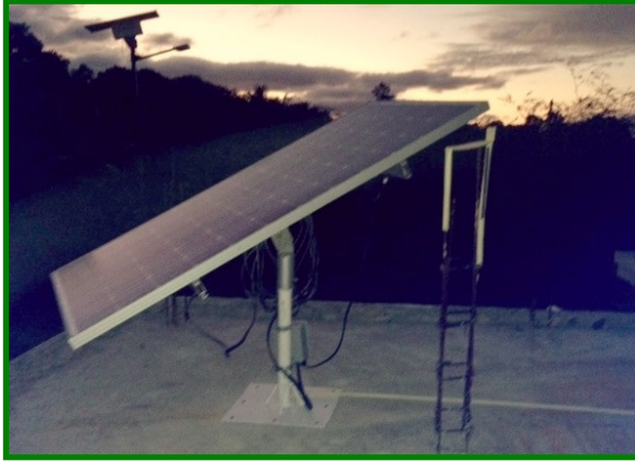
With joy you will draw water. (Is 12:3). The solar panel which powers the water system for Pilette.
